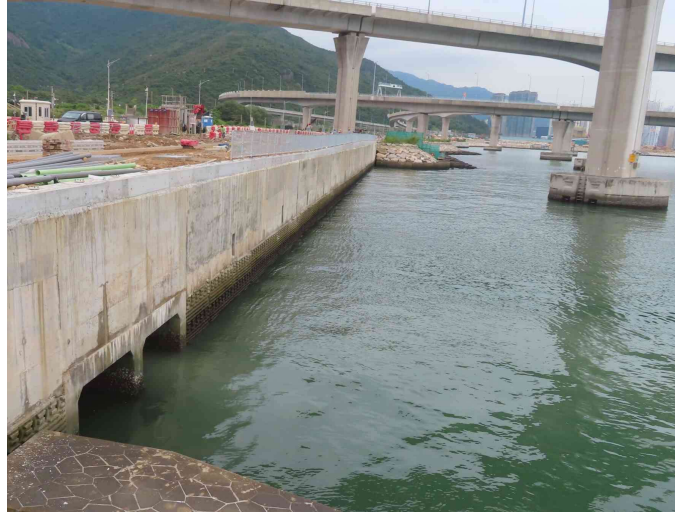
General View of Vertical Eco-shoreline
